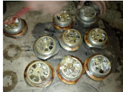
Figure 7 - Contaminated nozzles (Wärtsila Moss scrubber unit)
