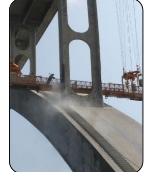
Krk: optical sensors embedded into columns
