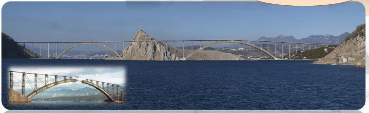
Krk bridges 1967-1980 RC arches 244+390 m innovative procedure forming a trussed arch cantilevers
