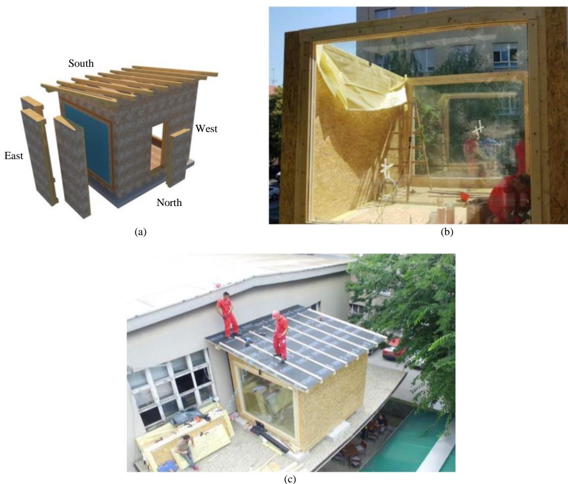
Fig. 6: Assembly process for the Live-Lab facility at the University of Zagreb, Croatia (installation during 2018): (a) general concept; (b) CLT-glass facade elements and (c) roof
