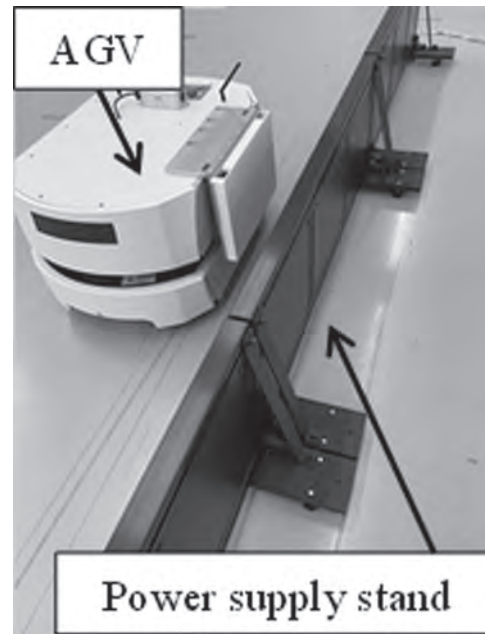
Fig. 1. Image of power supply to operating AGV
