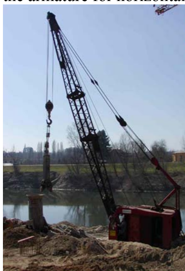
Fig. 17. Implanting pilots
