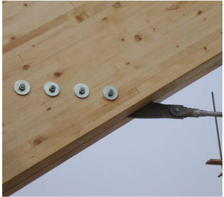
Fig. 10. Detail of connection of tie rod to main girder
