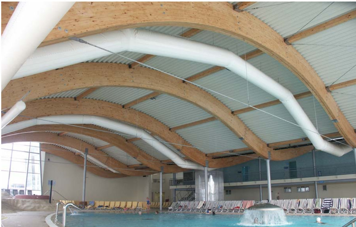
Fig. 11. Completed glulam structure with completely finished facility.
