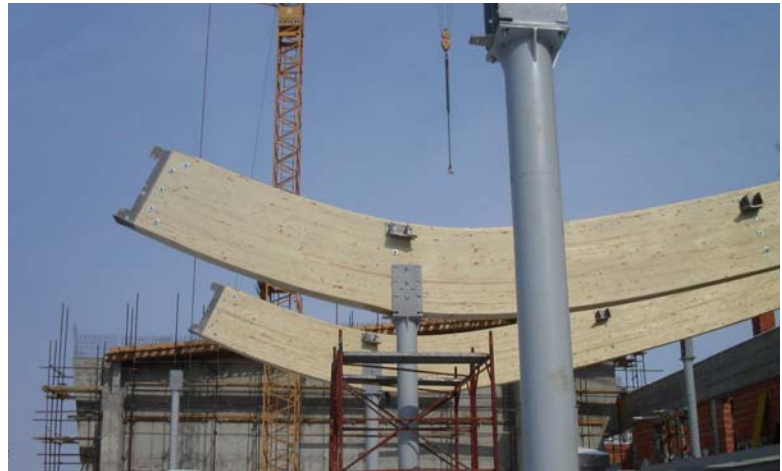
Fig. 7. Start of installation of main girders of the glulam structure
