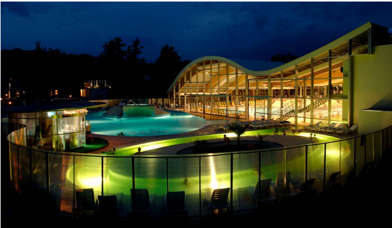
Fig. 12. Night view of the structure of roofed and open pools in St. Martin, Croatia
