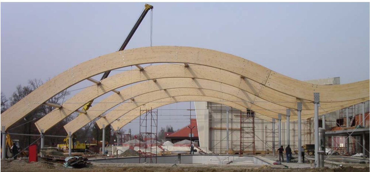
Fig. 8. Installation of timber structure in early April 2005.
