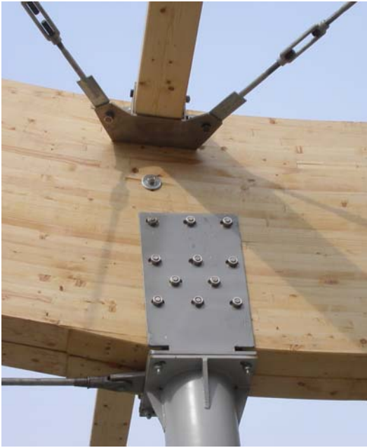
Fig. 9. Detail of support on central column
