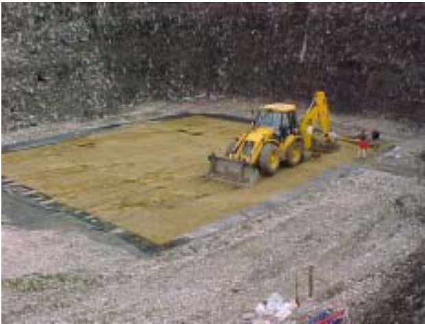
Figure 1. Investigation area inside the waste body
