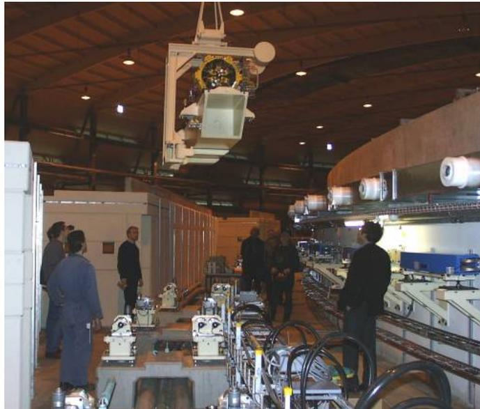
**Fig. 25:** Mounting of the first girder/magnet assembly onto its place in the SLS storage ring
