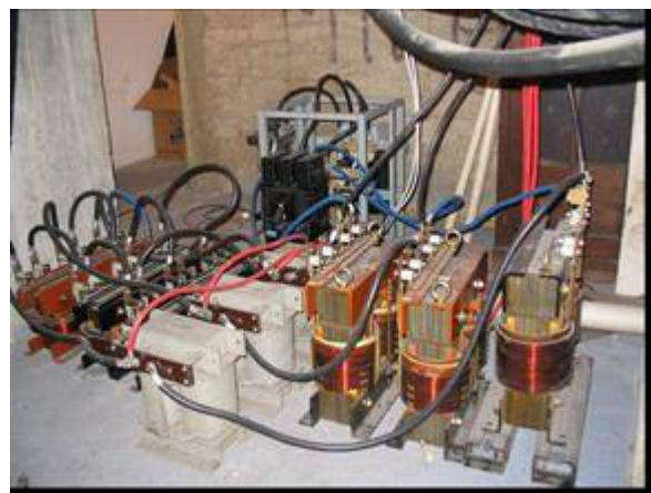
Fig. 9. Inductances used as parallel transmission lines
