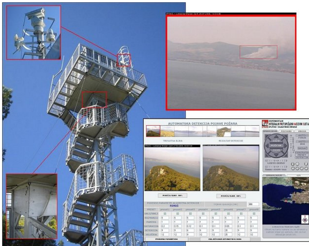
Figure 1. Croatian iForestFire monitoring station in experimental work on Marjan hill (Split area) during 2005 and 2006 fire season
