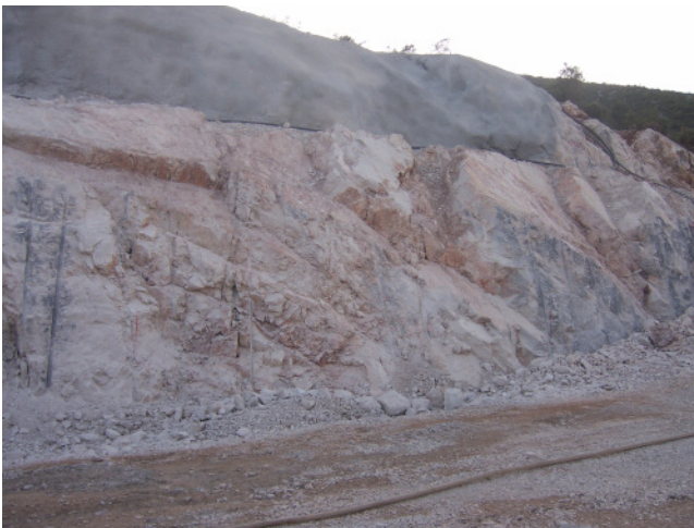
Figure 1. Bedding of rock mass dipped to the excavation face
