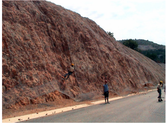
Figure 5. Slope protection with double twisted galvanized wire meshes
