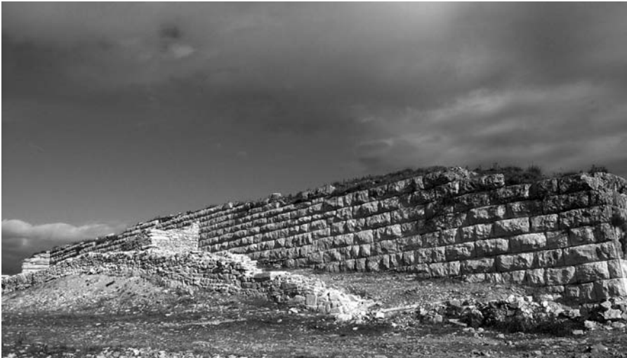
Fig. 1 - Asseria (Gradina near Podagra-Benkovac).
