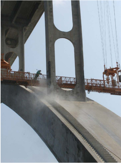
Figure 3: Removing of protective coat
