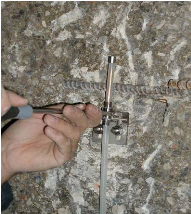
Figure 5: Sensor fixing onto inox bolts
