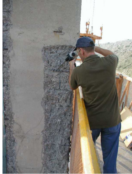
Figure 4: Flattening of concrete surface
