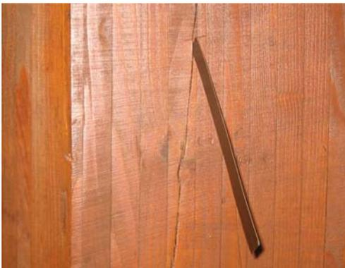
**Fig. 1:** Crack depth determination by thin plate penetration
