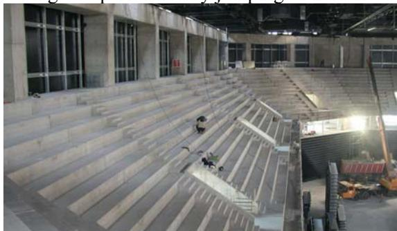
Fig. 5: Assembled grandstand structure.
