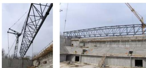
Figure 2: Lifting of complete roof truss by 500 t auto crane
