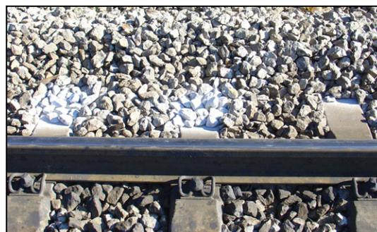
Fig. 2: Settlement of the concrete sleepers.
