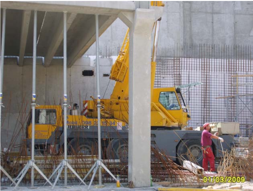
Figure 1: Completion of the precast construction depends on the completion of the monolith construction
