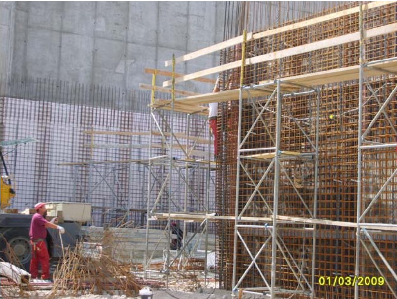
Figure 2: Completion of the stair case dictates the precast construction completion
