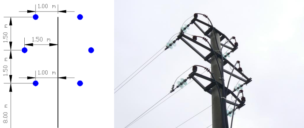
Fig. 3. Pole 1 of the double-circuit 10(20) kV overhead line
