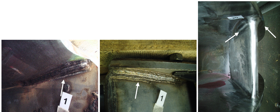
Figure 2. The welding repair and the changes in geometry by increasing the curvature radius
