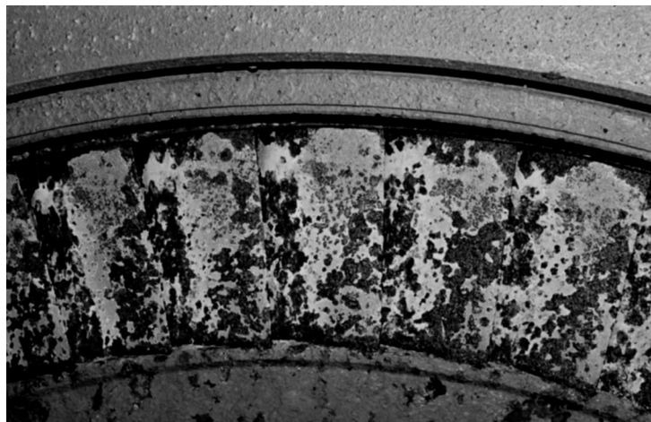
Figure 3. Severe corrosion of stationary turbine blades
