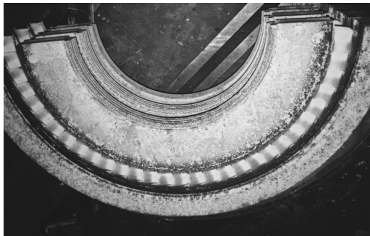
Figure 2. Corroded distribution walls with stationary blades
