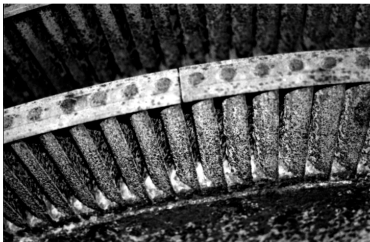
Figure 5. Severe corrosion of turbine moving blades profile
