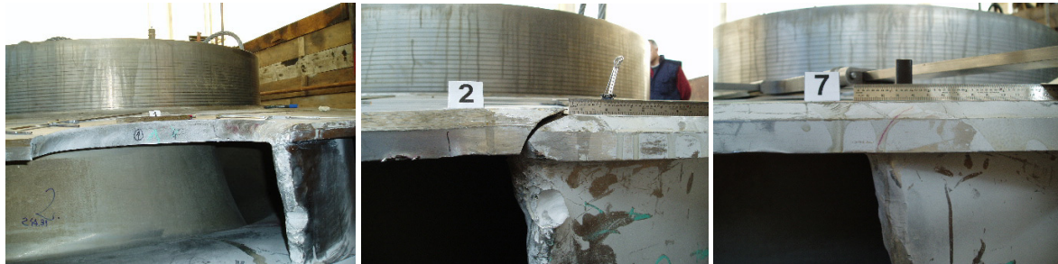
Figure 1. The turbine rupture
