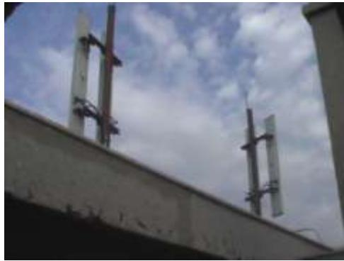
Figure 5. A view to two sectors of the base station antenna system
