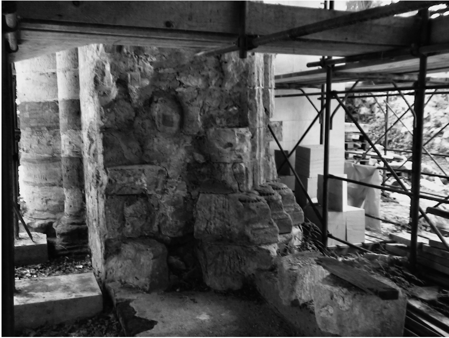
Fig. 4. Topusko, detail of the church portal. (author, 2010)
