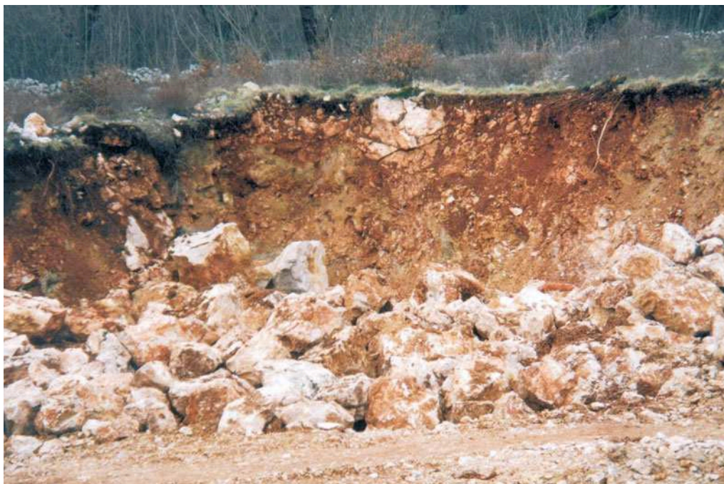
Figure 5.31. Till (MDcmm lithofacies) exposed by construction works beside the road to Malinska. Many metre-sized and even larger boulders were left in piles. Some ice-faceted and ice-polished boulders were found. Besides coarse-grained matrix, locally appears clayey matrix of greenish-gray color (see figure below). Photo taken in 2003.
