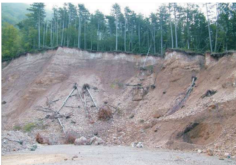
Figure 3.22. Pleistocene stratified coarse to fine gravels exposed in a gravel pit near Vratnik K(SD)-10. Photo taken in 2008.
