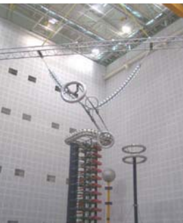
Fig. 6. E: 400 kV "V" suspension glass insulator string
