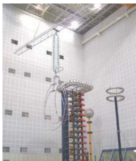
Fig. 7. F: 400 kV double tension glass insulator string
