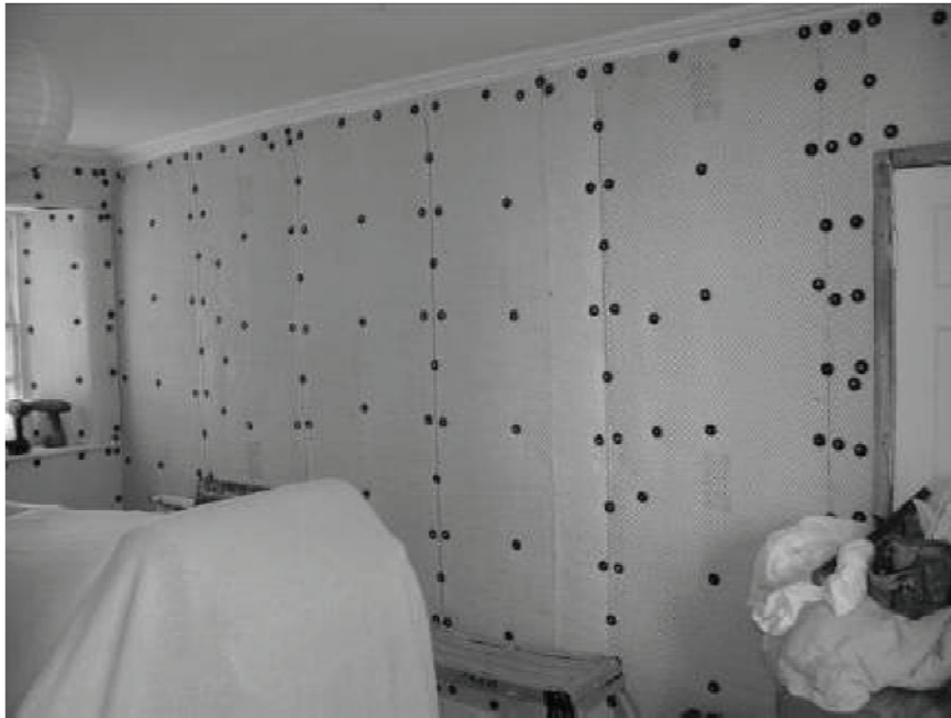
Figure 5. Application of a thin aerogel matt. Note the cornice is unaffected.
