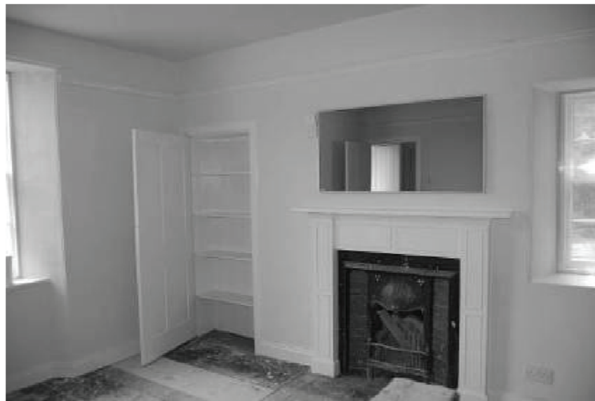
Figure 7. Radiant heat panel (the “mirror” above the fireplace) being trialled in a rural cottage.
