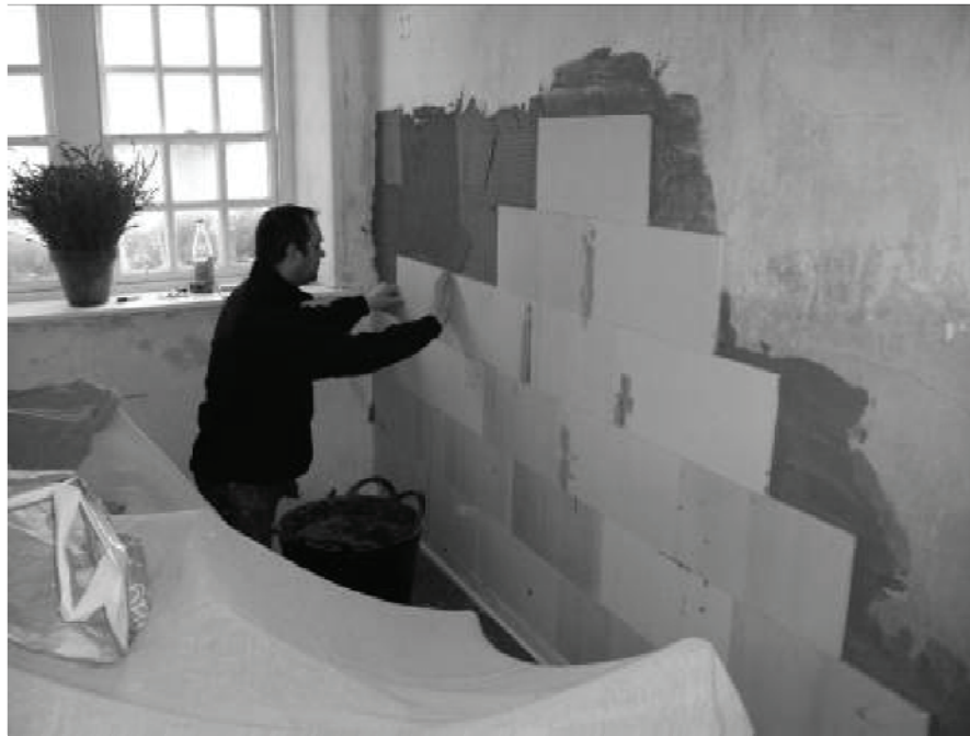
Figure 6. Application of calcium silicate board to an existing plastered surface.
