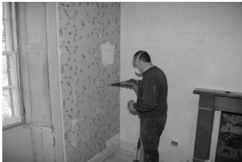
Figure 4. Application of blown cellulose insulation (Historic Scotland).
