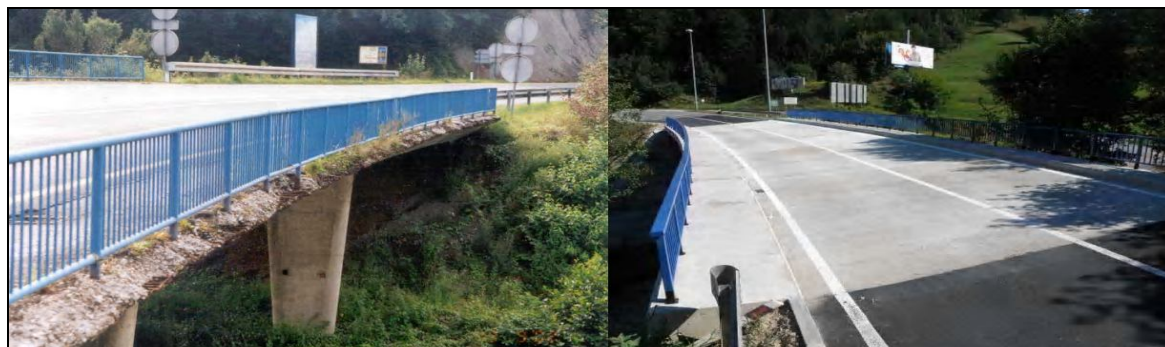
Fig. 1 Macelj Overpass before and after rehabilitation
