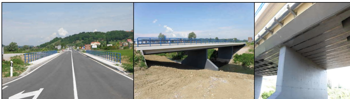
Fig. 3 Reconstructed bridge with details of strengthening by fiber reinforced polymer
