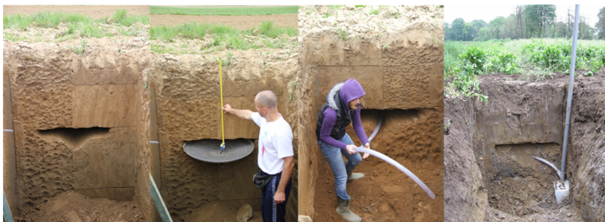
Figure 2: Stages of the field lysimeters installation
