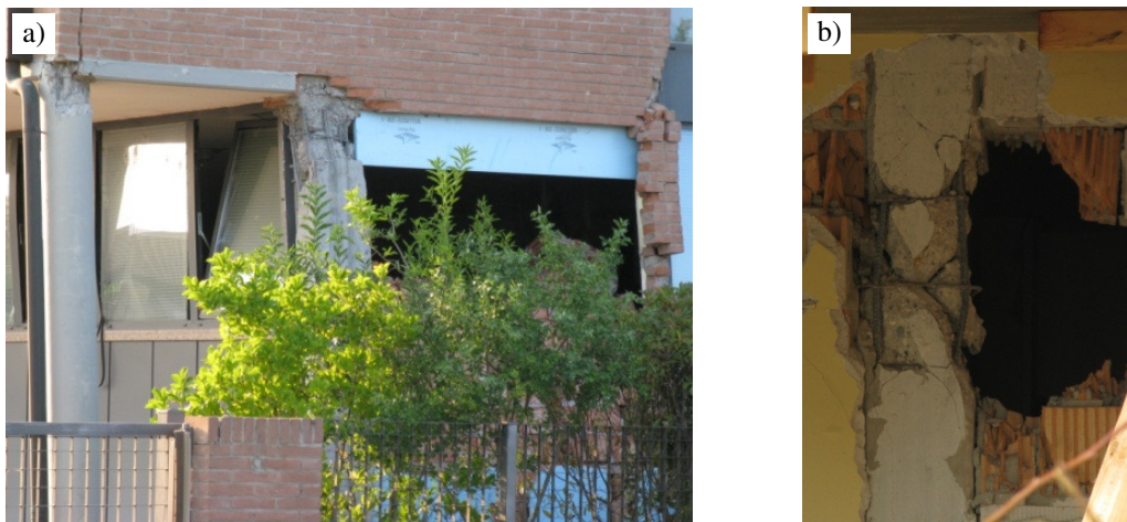
Figure 1: Examples of local effects reported after the May 2012 Emilia earthquake a) Magenes et al. 2012 [3]; b) Manzini and Morandi 2012 [4].
