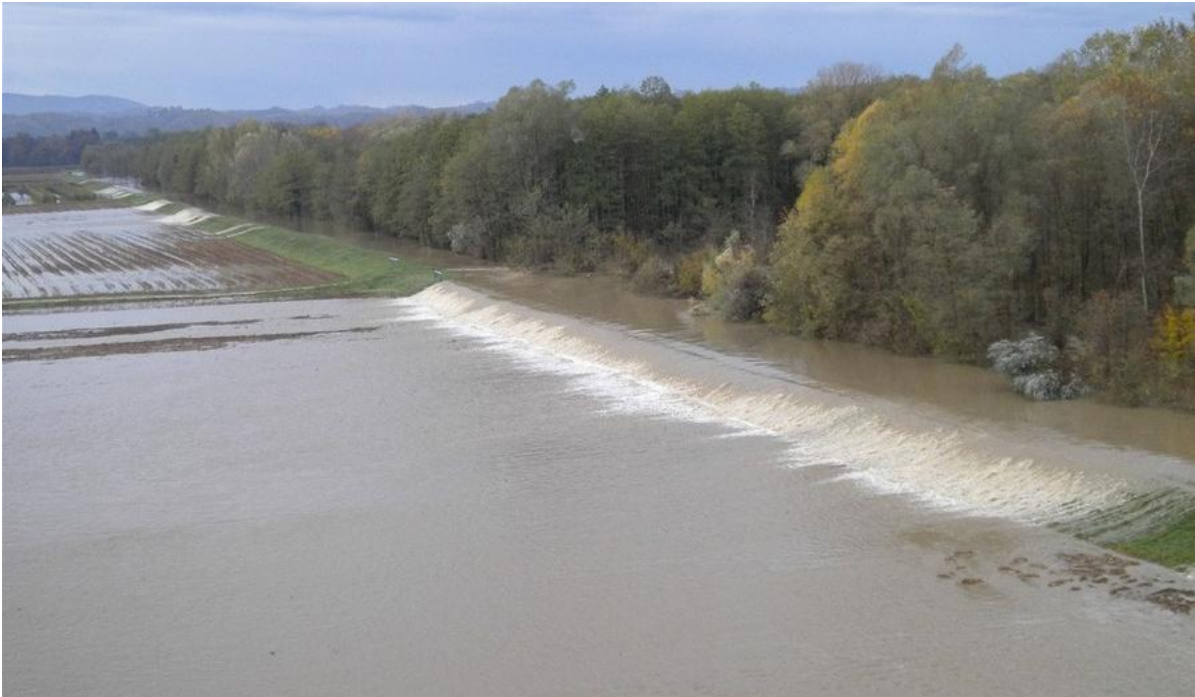
Fig. 18 Over-spilling of the Virje Otok-Brezje levee (time unknown, source Internet)
