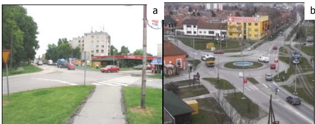
Figure 3: Vinkovačka-Drinska St. intersection – before and after the reconstruction
