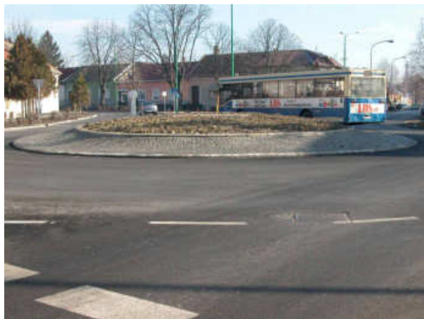
Figure 1: Roundabout after the reconstruction (2005)
