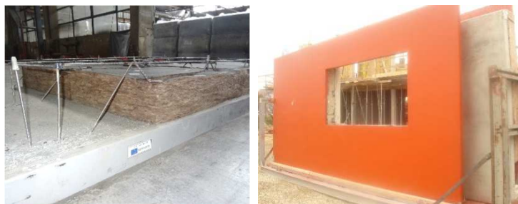
Figure 6 Production and transportation of ECO-SANDWICH® to the construction site
