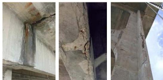
Figure 4. Deterioration of Adriatic bridges
