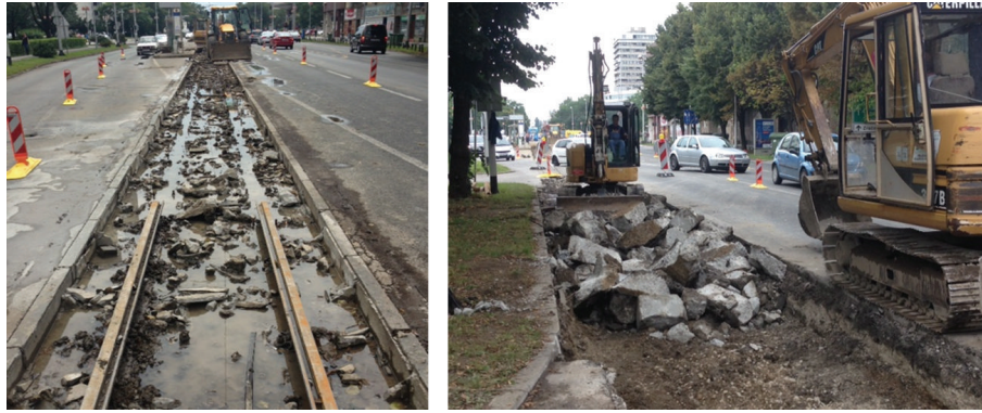
(a) Demolition of existing tram track
