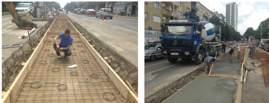
(c) Fitting strain gauges to slab reinforcement (left), casting of new reinforced concrete slab (right)
