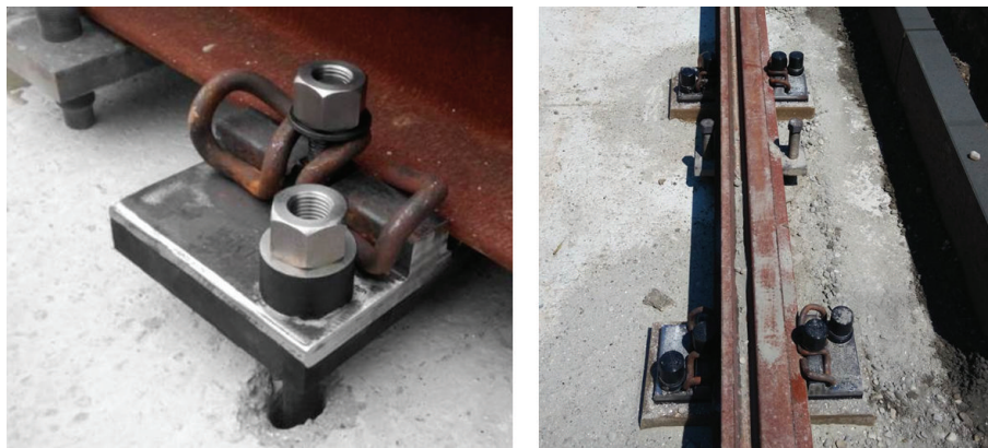
(b) Construction of the levelling layer with 2I-CTT fastenings and rail mounting
