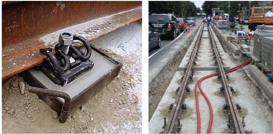
(a) Construction of the levelling layer with PPE fastenings and rail mounting
