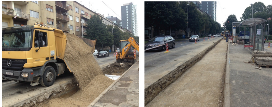
(b) Construction of the new mechanically compacted base layer
