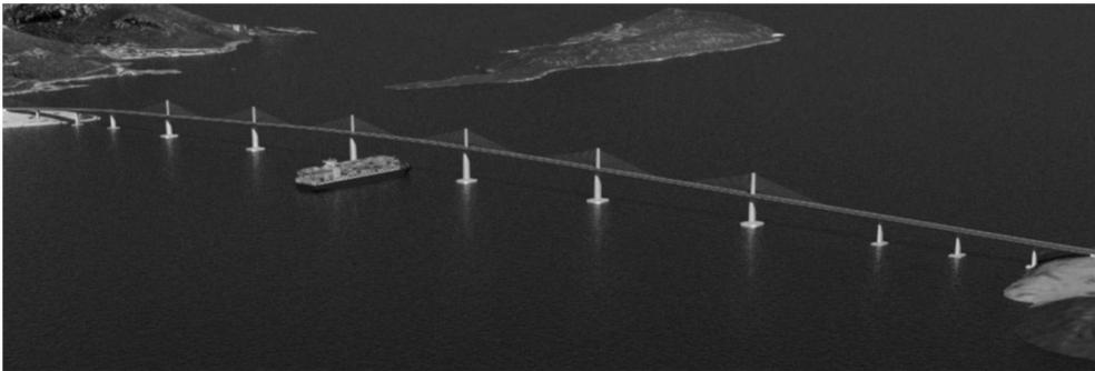
Figure 9. Computer rendering of multi-span semi-integral extradosed bridge – aerial view.
