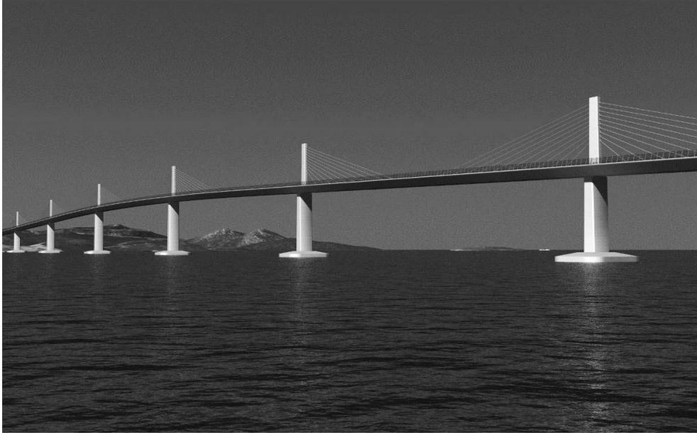
Figure 10. Computer rendering of multi-span semi-integral extradosed bridge – close-up view.
