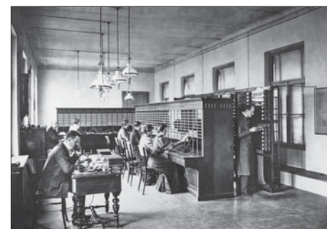
FIG. 24 C.B. TYPE SWITCHBOARDS IN THE TELEPHONE HALL AND MANUAL OPERATORS
