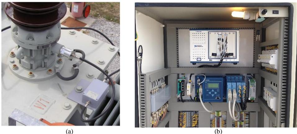
Fig. 1. (a) Connection to measuring tap; (b) Transient overvoltage monitoring system (Končar TMS+) installed on shunt reactor
