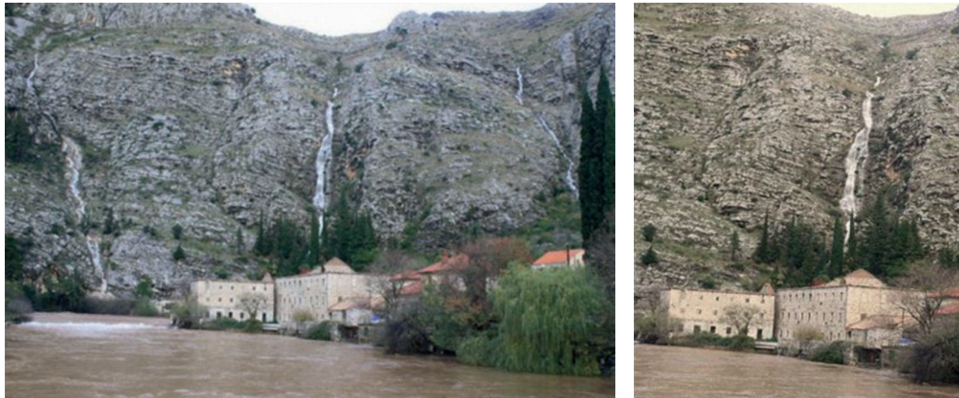
Fig. 10 Water level in the underground reservoir in a specific situation of high water levels in the spring zone (November 2010.)
