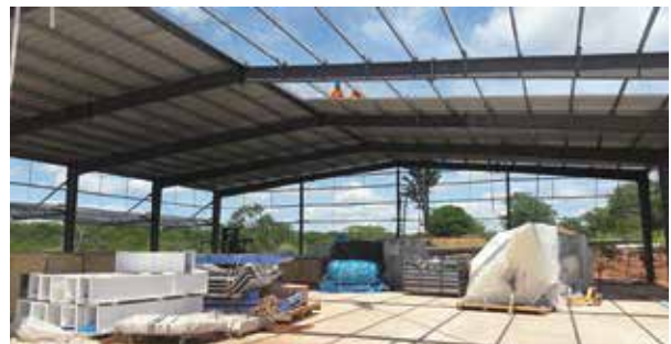
The Zambian factory under construction, February 2017
