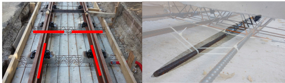
Figure 5. Position of strain gauges prior to concrete casting on 21-STT subsection.
