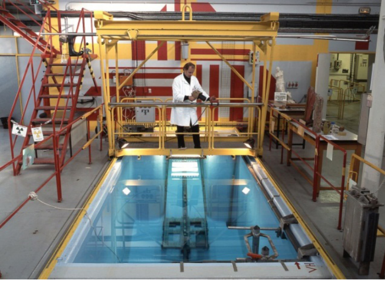
FIG. 26.1. The ARC-Nucléart irradiation facility.
