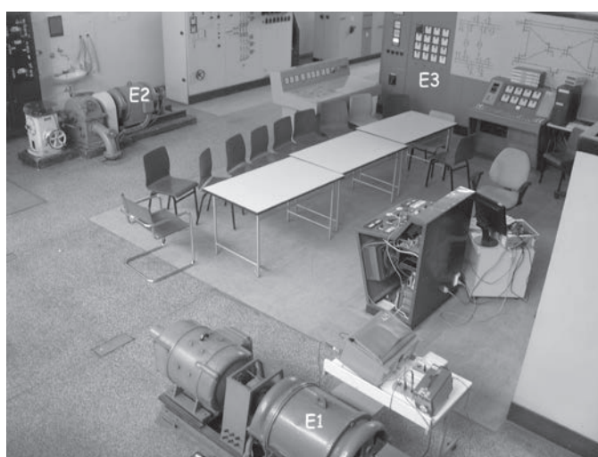
Figure 1. Part of power system laboratory
