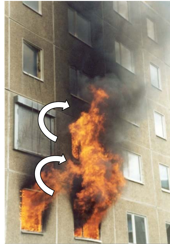
Figure spreading of fire across facade (Source: Khotoff, 2015)
