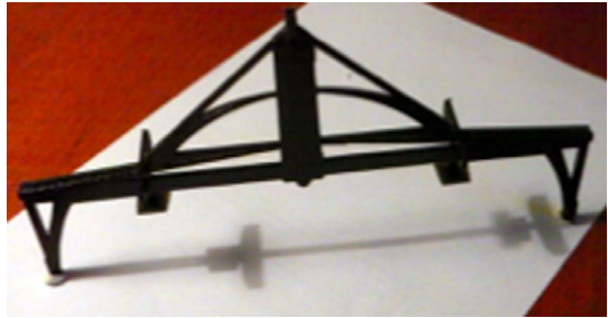
Fig. 4. A rapid prototype of a wooded roof truss, part of the structure damaged badly in the recent fire at the Mackintosh School of Architecture at the Glasgow School of Art
