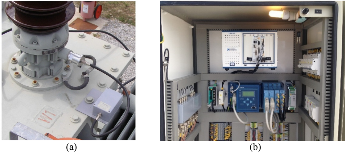
Figure 3. (a) Connection to measurement terminal of bushing; (b) Transient overvoltage monitoring system (Končar TMS+) installed on power transformer
