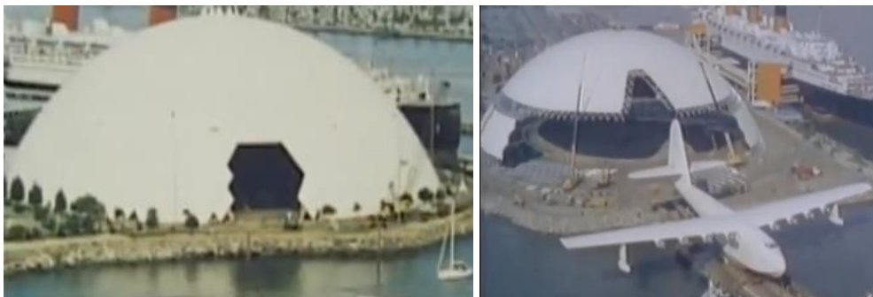
Figure 2: Spruce Goose Dome, Long Beach, California
