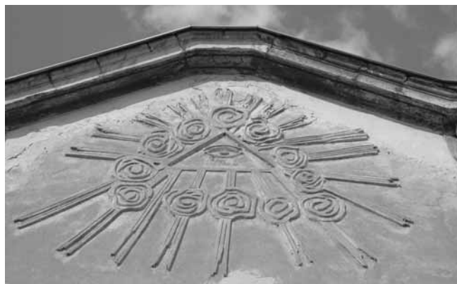
7. Štuko amblem s prikazom Božjeg oka na zabatu pročelja. Stucco emblem depicting 'The Eye of God' on the façade pediment.
