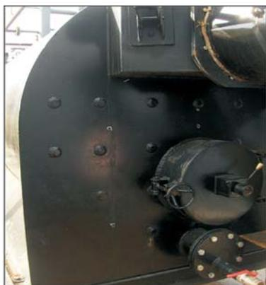
Figure 1 Measurement points along the boiler rear head
