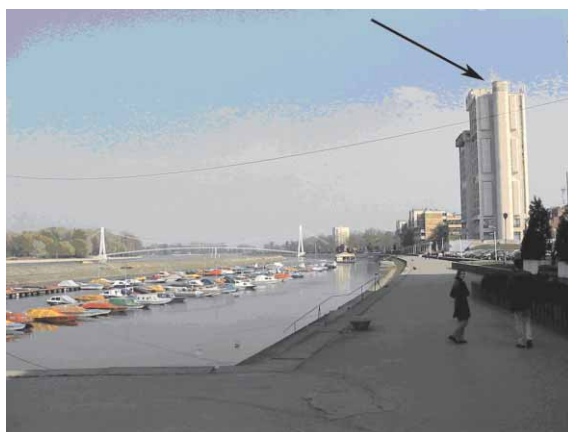
Figure 1. View of the monitoring site (from west to east) where the instrument was placed near the roof of Hotel Osijek, as indicated by the arrow.
